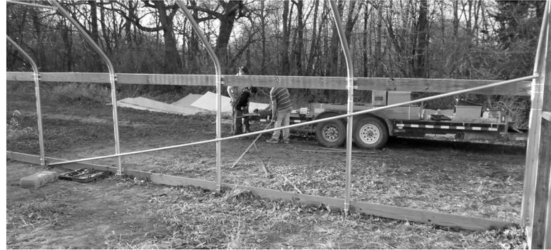
Purlin pipes run the length of the frame inside the arches, always one at the peak and generally 1-3 on both sides. Always fasten the Purlin pipes at the peak and top of straight side with pipe straps and three #12x1" Tek Screws because cross connectors will tear the plastic with time.
